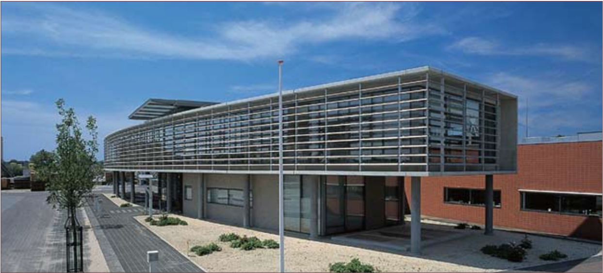
External Horizontal Custom Louvres - Commercial office library
