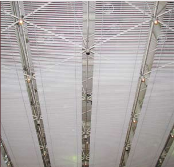
Ceiling Rack Arm System - National Gallery of Australia, Canberra
