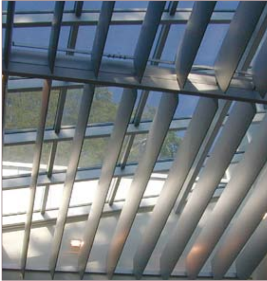
Louvres fixed within a glass roof
