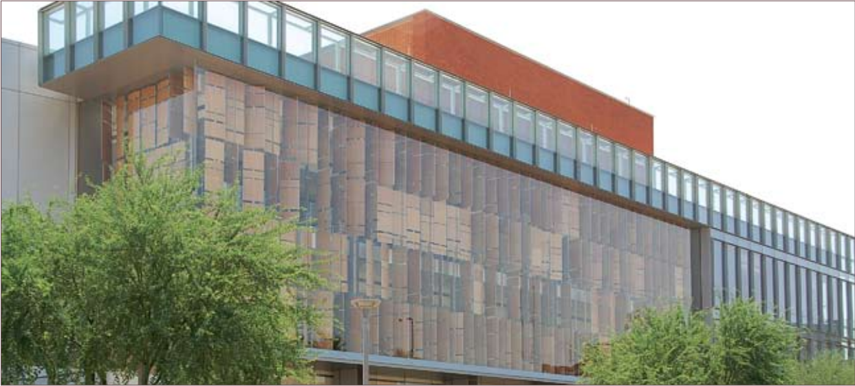
Custom made Speciality Wood Louvres in double-skin facade - Biodesign Institute, ASU
